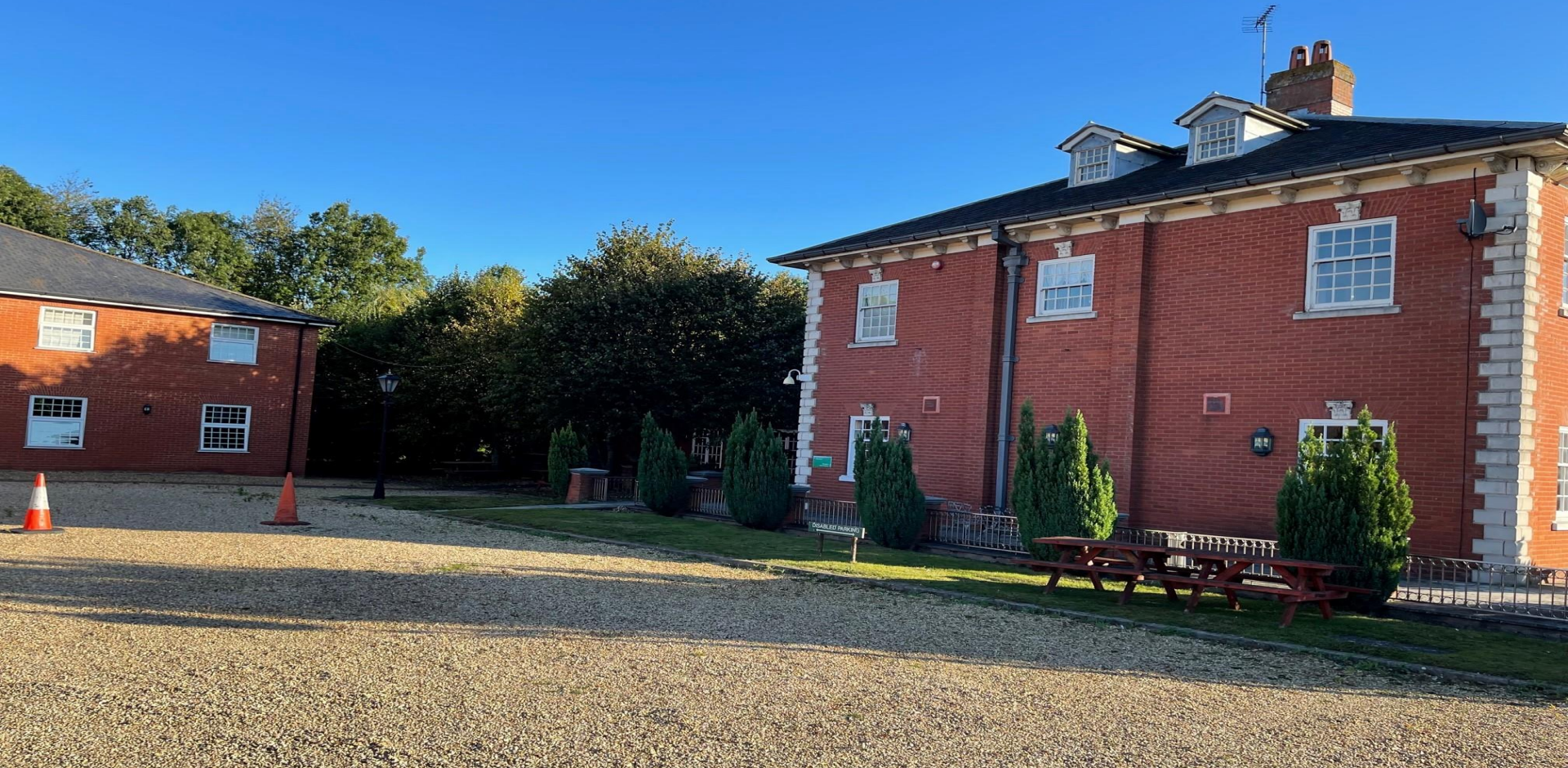
Hotel to east of application site
