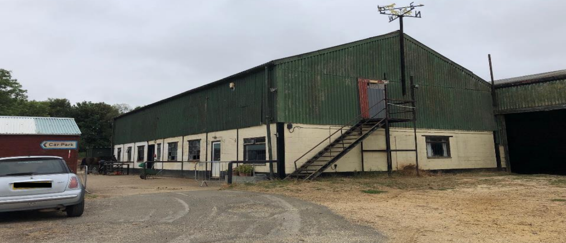
View west of application building (right) and livery building (left)
